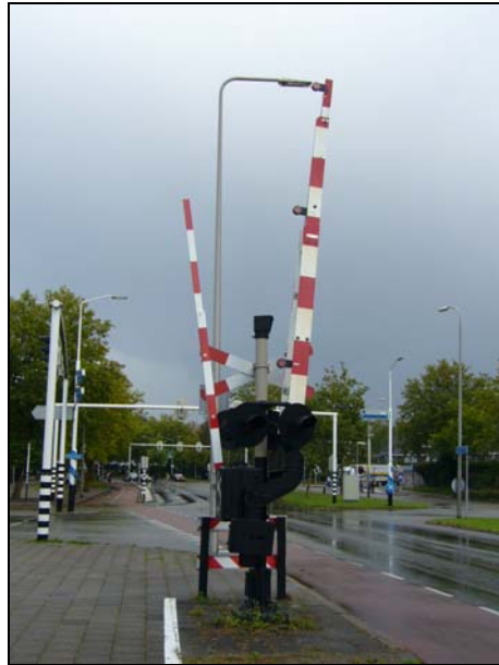
Photo 4: Level Crossing barriers.
