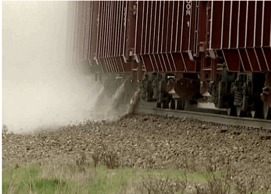
Picture 4: 'Plus Train' Unloading Ballast at Circa 30kph
