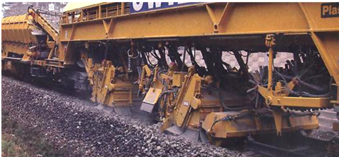
Picture 5: BDS Sweeper Unit Picking-up Excess Ballast for Redistribution
