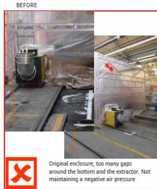
Isocyanate paint spraying in train carriage refurbishment
